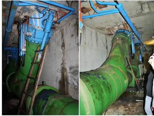
**Figure 10.** Branches to the turbine unit.
