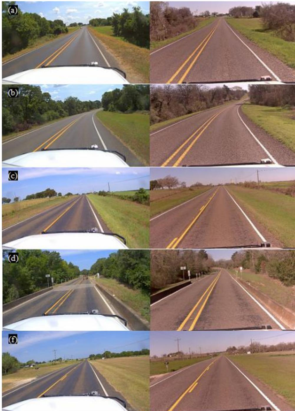
**Figure 5.** Case III Surface Conditions: Before (Left) and After (Right) Chip Seal at (a) EB 2095 ft – Slightly Flushing after Chip Seal, (b) EB 5 ml 3257 ft – Slightly Flushing after Chip Seal, (c) WB 4488 ft – Flushing after Chip Seal, (d) WB 2 ml 495 ft – Flushing after Chip Seal, (e) WB 4 ml 1531 ft – Flushing after Chip seal, and (f) WB 7 ml 422 ft – Flushing after Chip Seal.
