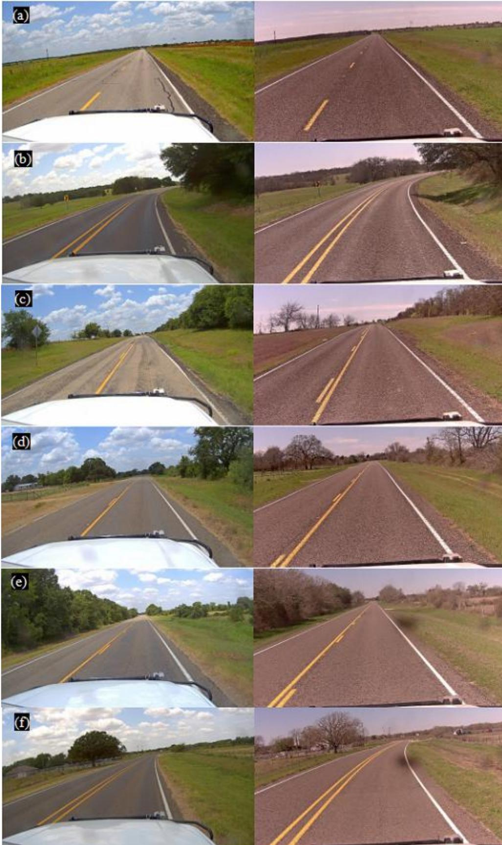
**Figure 4.** Case II SB Surface Conditions: Before (Left) and After (Right) Chip Seal at (a) 4439 ft – Slightly Dry/Rock Lost after Chip Seal, (b) 2 ml 2736 ft – Dry/Rock Lost after Chip Seal, (c) 5 ml 1811 ft – Dry/Rock Lost after Chip Seal, (d) 9 ml 3115 ft – Good after Chip Seal, (e) 11 ml 2904 ft – Good after Chip Seal, and (f) 12 ml 3683 ft – Good after Chip Seal.
