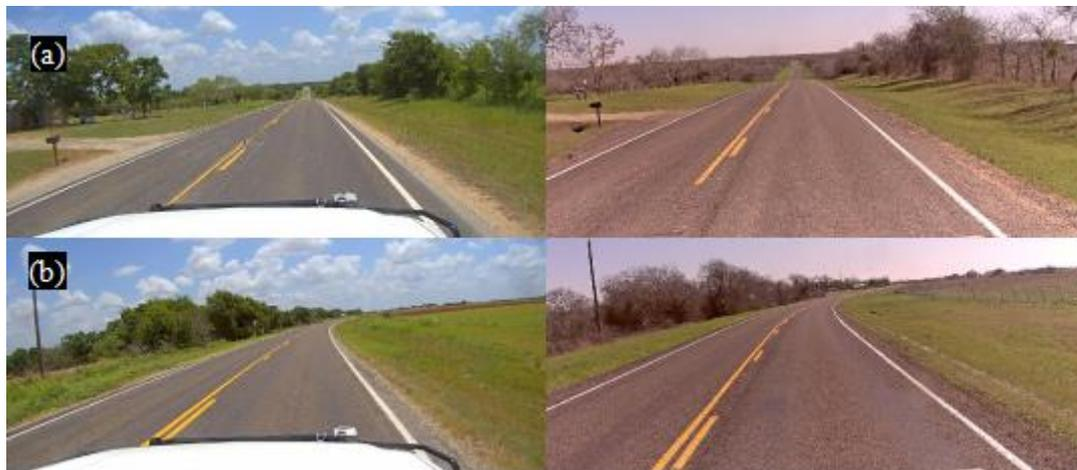
**Figure 3.** Case I EB Surface Conditions: Before (Left) and After (Right) Chip Seal at (a) 1 ml 2230 ft – Slightly Dry/Rock Lost after Chip seal and (b) 2 ml 537 ft – Slightly Flushing after Chip Seal.
