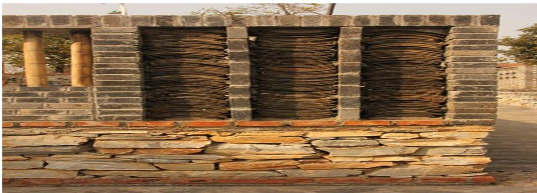
*Figure 5. A wall built with black bricks, black tiles, stones and bamboos.*
