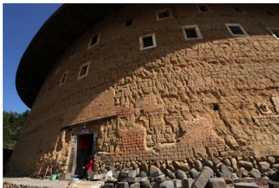
*Figure 5. Rammed Soil Wall Structure of Earth Building.*
