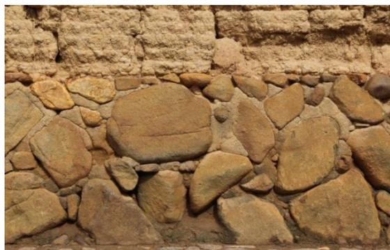
*Figure 4. Stone foundation of Earth Building.*
